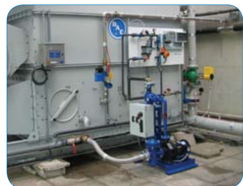
Filter Installation
