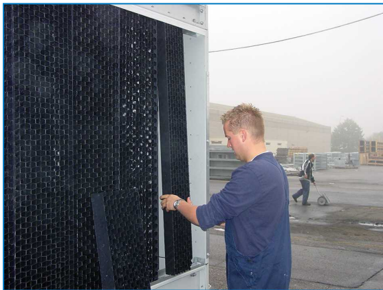
Remove combined inlet shields
