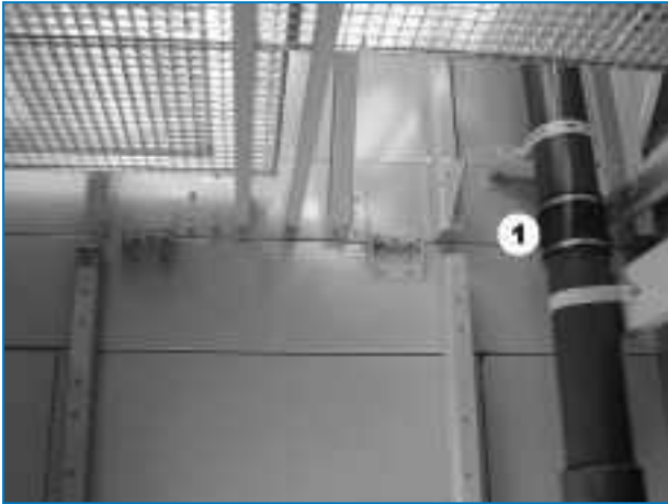
Sleeve with hose clamps
